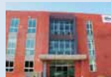
Peking, China ○ IGBT-Stack-Montage
